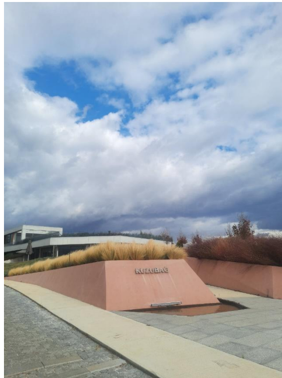
Photo 2. Kuzubağ Winery: Construction in line with the landscape
