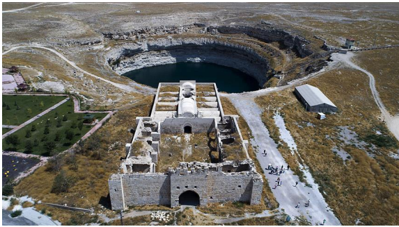
Figure 4. General View of the Kızören Sinkhole (www.aa.com.tr)
